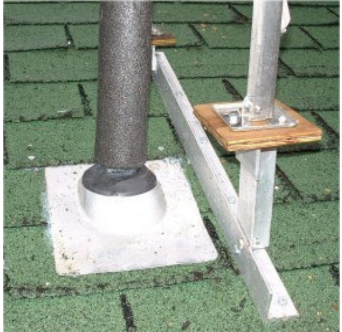
Detail of roof penetration
